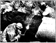
**8** Welding – the work here assumes use of automatic welding to join the sections of line pipe, which provides consistency, uniform welds and fewer repairs. To prepare the line pipe for automatic welding, a beveling and facing machine trims, cuts and grinds the pipe ends with the special edge preparation required by the process. Line pipe comes from the pipe mill with a standard edge preparation or with a plain end if the pipe is specially ordered for automatic welding.
