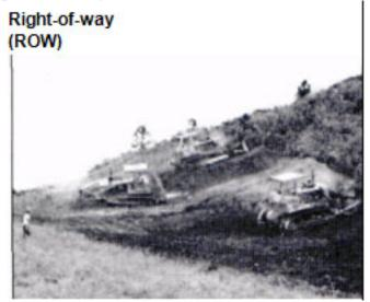
*3 Ditching* – excavated soil (*spoil*) is deposited on the ditch bank. In certain areas, particularly farmland, the ditch will be excavated in two passes with a first pass removing *topsoil* and the second *pass* excavating the remaining soil to the required pipeline *burial depth*.
