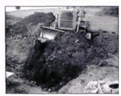
**17 Final clean-up, ROW restoration** – grading the ROW smooth and clear, placing marker signs to identify the pipeline location, repairing any fences or other structures temporarily removed for construction and seeding the soil to reintroduce vegetation are the final activities. Special attention is paid to drainage and erosion control so that ROW, with time, is restored as closely as possible to its pre-construction while allowing access for regular visual inspections.
