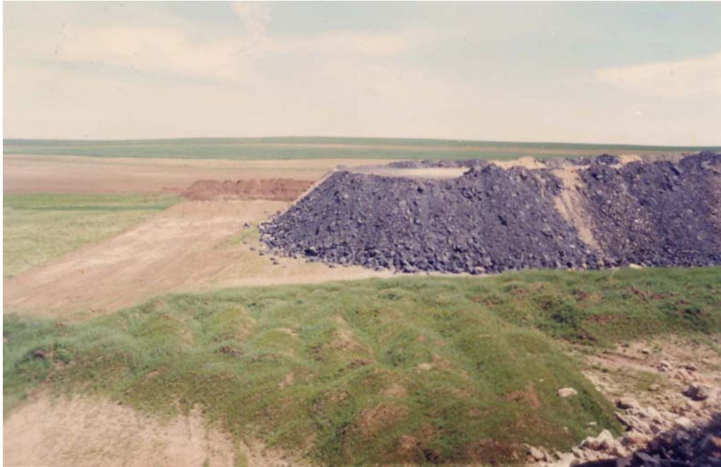
Fig. 53. External dump of waste rocks at «Chalpan» area of Vostochno-Beysk coal open-pit mine.
