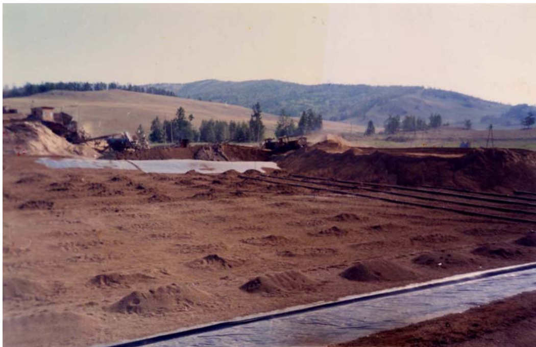
Fig. 44. Heap base laying. The base is covered with special durable polymer material (light) preventing from cyanide into underground waters
