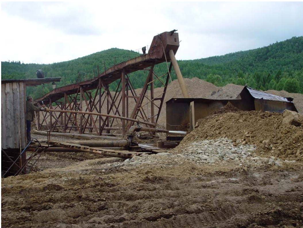
Fig. 26. Washing unit on river Andat
