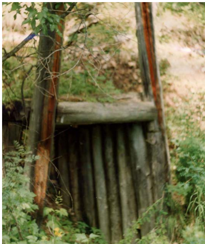
Fig. 31. Exploring gallery entrance at Ipchul Cu-Mo field
