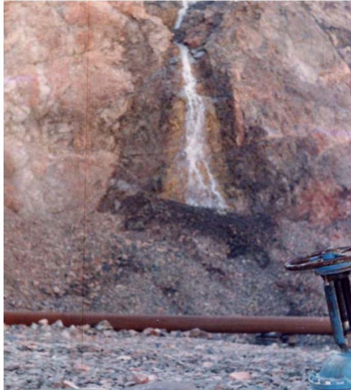
Fig. 39. Head fracture water in the quarry of Sorsk field. Pumping down from the quarry is performed along the piping system
