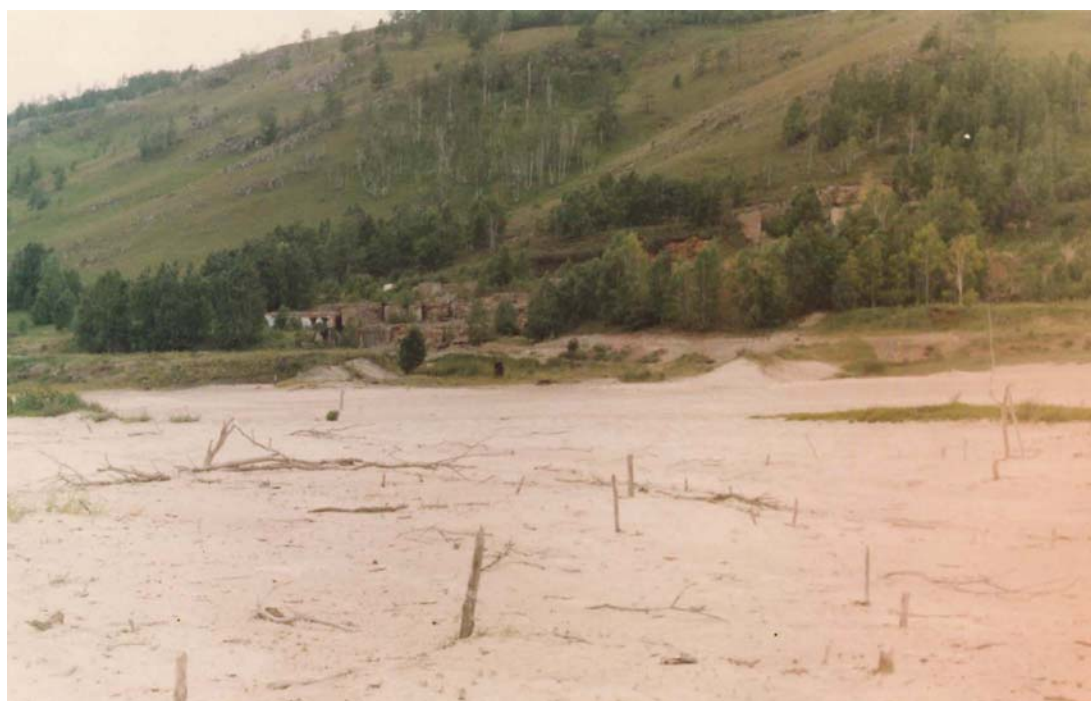
Fig. 35. Old tailings dump of Julia field makes possible wind ablation of harmful chemical elements. At the background there the remains of the concentration plant
