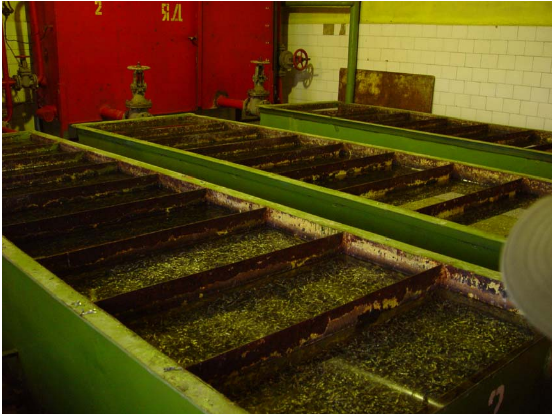
Fig. 48. Reservoirs with zinc shavings for gold precipitation from solution
