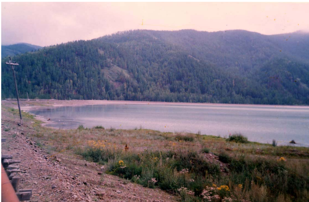
Fig. 61. Sediment tank of cyanic solutions at Kommunar field
