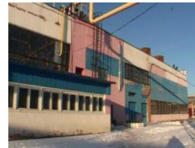
Local boiler plant
