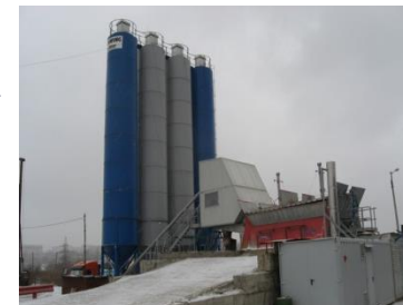
reinforced concrete plant
