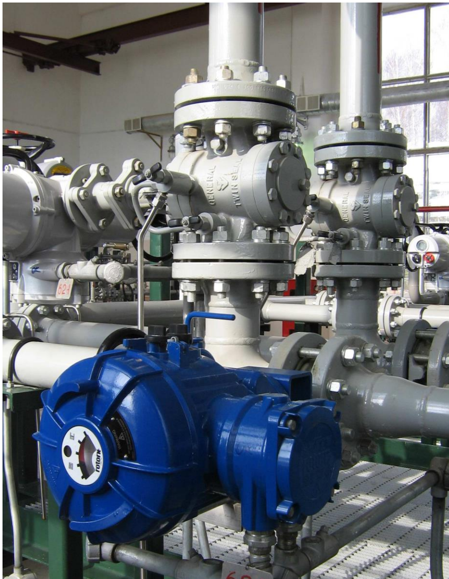
Fig. 4.19. Control flow valve- FCV
