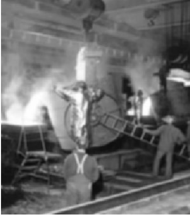
Figure 9: Steel-making machinery [wikipedia]
