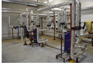
Individual heating substation
