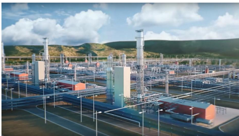
Figure 1.3 Advanced development zone «Svobodny»
